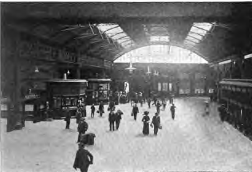
ASSEMBLY PLATFORM, ADELAIDE RAILWAY STATION.
